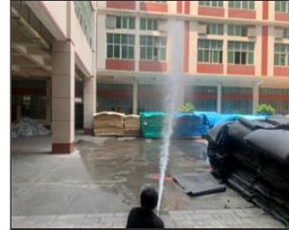
External photo(s) of the production unit(s) Testing of fire hydrant.JPG
